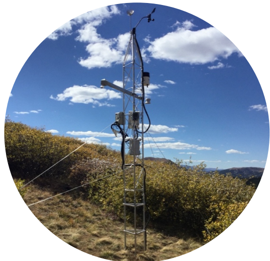
The new tower at Independence Pass. Image Credit: Elise Osenga
